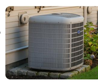
Heat pumps with inverter-driven or multi-speed compressors offer variable output to cater to large temperature variations, maintaining continuous comfort. Single-stage heat pumps operate more like traditional systems as they do not vary their outputs. Understanding how to operate and maintain your heat pump can enhance energy savings and cost efficiency. Review the provided tips, FAQs, and contractor advice to optimize your heat pump's performance.
